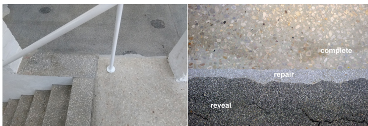
Fig. 5. polished concrete floors in the MAD building (a+b: Melanie Tamm, 2016)
