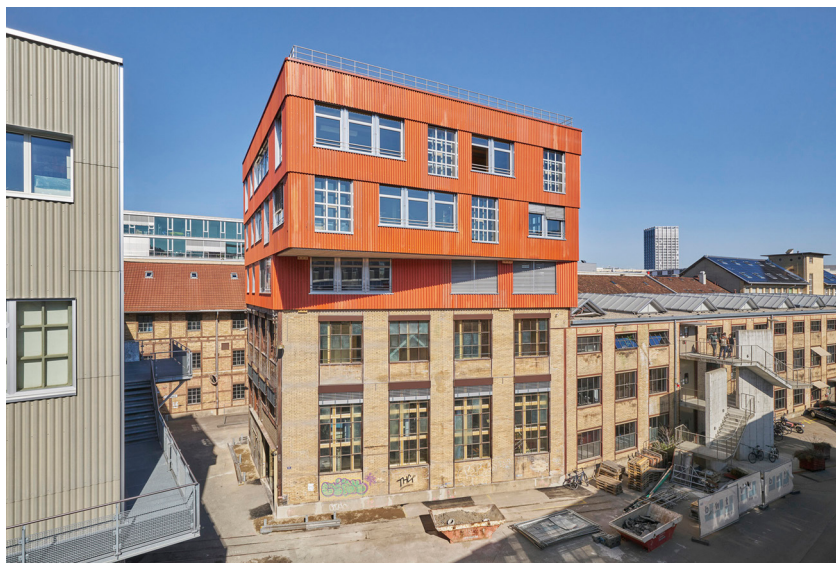
Fig. 3. The Facades of the Extension and the Existing Building in K.118 Project, Winterthur (Martin Zeller, 2021)
