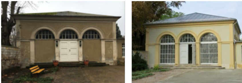
Fig. 1 Original and new facade
