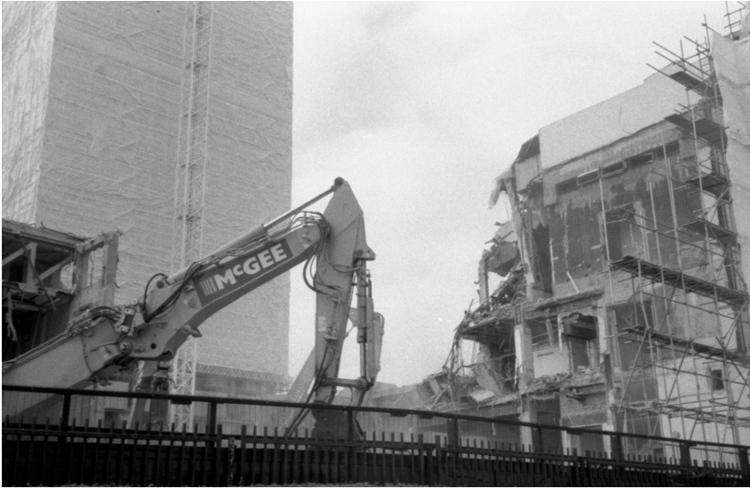
Fig. 1. Demolition and rehabilitation site, London (Paul Susini, 2025)
