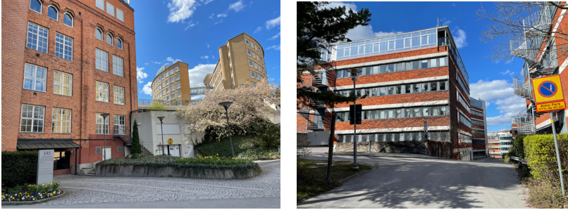
Fig. 2. Left. To be retained: A former factory in the foreground with postwar “banana buildings” in the back. Fig. 3. Right. Due for demolition: Plot B’s 1980s office buildings (Cecilia Sundström, 2025)
