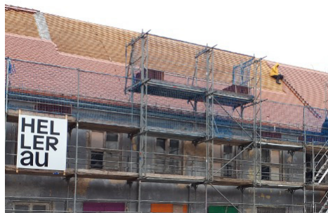
Fig. 4. Removing roof tiles for re-use (photo by Heinlewischer, 2022)
