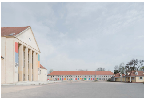
Fig. 1. View of the Festspielhaus Hellerau (left) and the east wing before renovation (photo by Brigida González, 2019)
