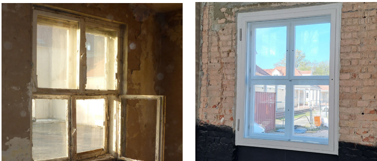
Fig.3. Casement windows before and after renovation (photos by Heinlewischer 2018, 2022)
