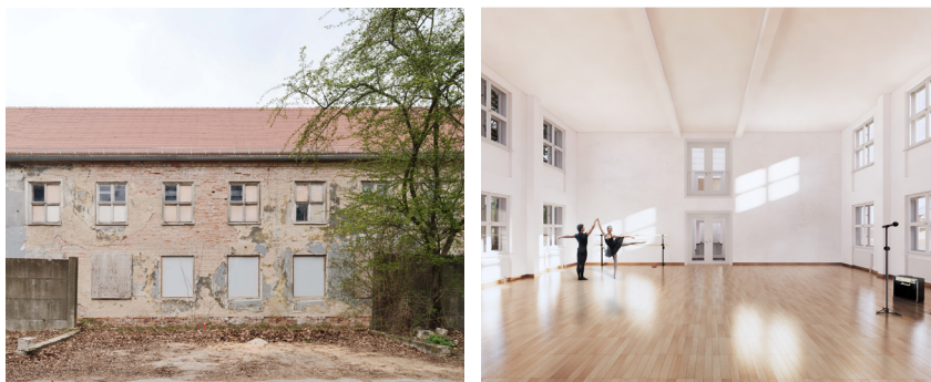
Fig. 2. East façade before renovation and visualisation of the rehearsal stage (photo by Brigida González 2019, visualisation: heinlewischer, 2020)
