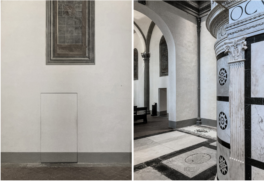
Fig. 3.1 (Left) and 3.2 (Right). The new opening in the wall reconnecting the chapel with the museum (Vanni Sacconi, 2025)
