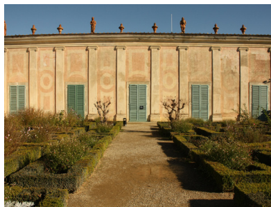
Fig. 2. The Palazzina del Cavaliere, one of the least accessible points of the garden, where the Accessibility Plan identifies a point of least resistance for the installation of a new elevator (Mirko Romagnoli, 2022)
