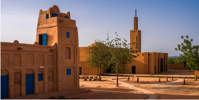
Fig. 2. Hikma Community Complex (James Wang, Courtesy of Mariam Issoufou Architects, 2018)
