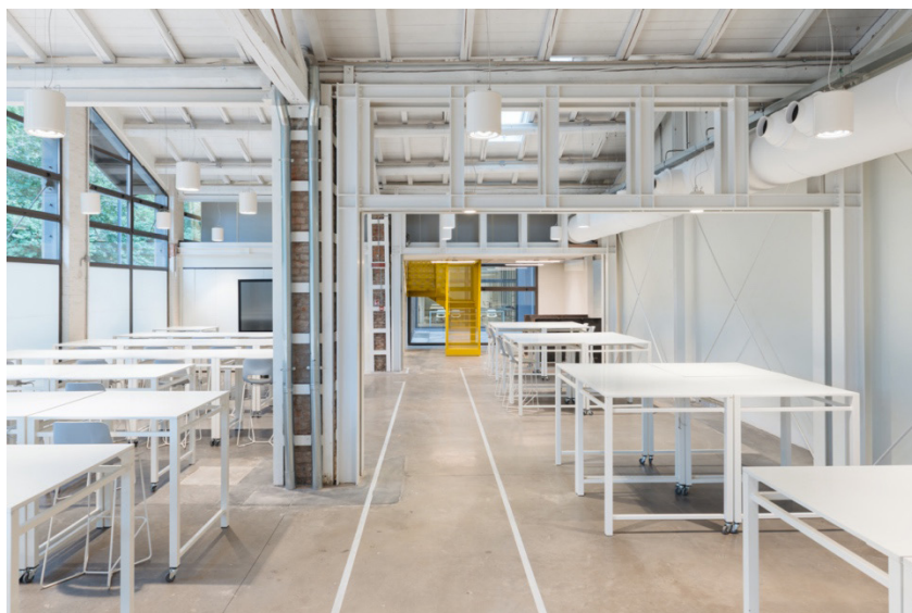
Fig. 4. The Learning Factory. Anti-seismic steel structures integrated with the architectural elements (Photo by Massimo Nicolino, 2020)
