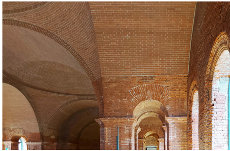
Fig. 1. Contemporary intervention in dialogue with the preexistence. Restoration of the vaults using traditional techniques integrated. Material discernibility not contrasted and analogous forms (photograph by the author).
