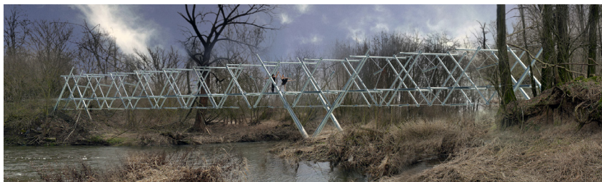
Fig. 1. Slup Tensegrity Footbridge (Petra Buganská, 2015)
