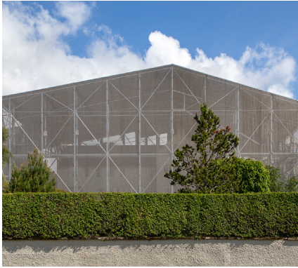
Fig. 1. Hill House Box (exterior). Carmody Groarke (Tom Parnell, 2019)
