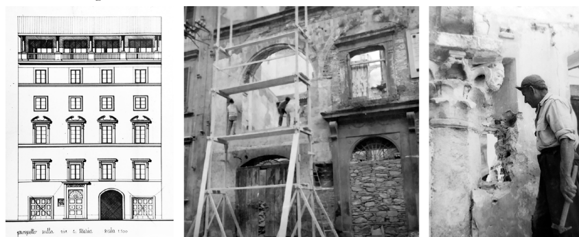
Fig. 2. At left, the refused façade design, 1958; At right, scraping and liberation of architectural elements ( Archivio Generale, SABAP-PI , f. 120, m. 231)
