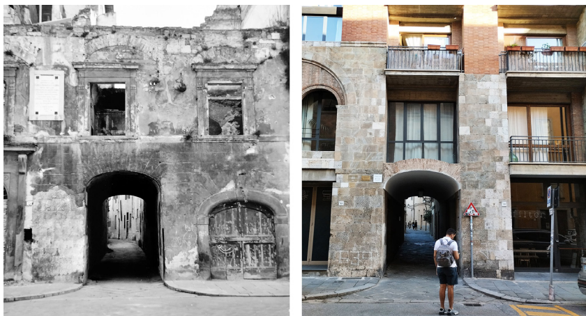
Fig. 1. At left, view from the Santa Maria Street, c. 1950s ( Archivio Generale , SABAP-PI, f. 120, m. 231); At right, current condition of the building (Pedro Freitas, 2024).
