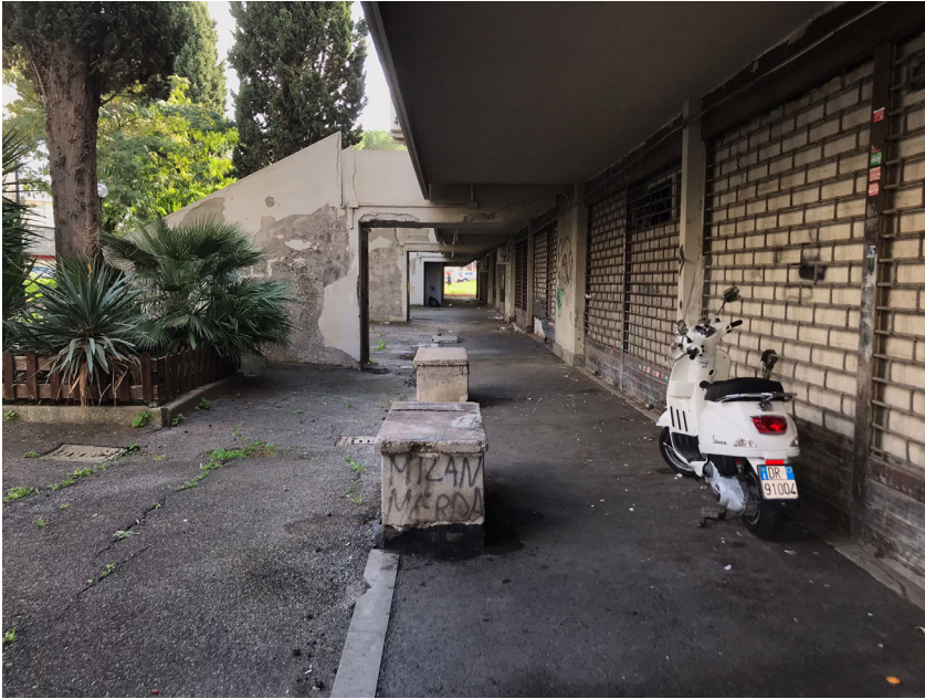
Fig. 2. Closed shops on the ground floor of the houses (Milena Farina, 2025)
