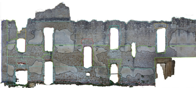
Fig. 1. Semantic segmentation according to homogeneous portions of masonry
