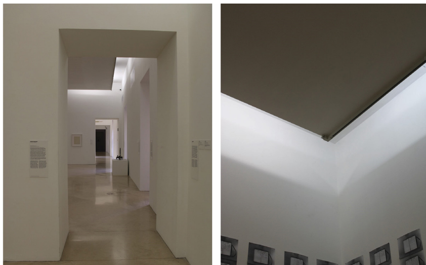
Fig. 3. Interior exhibition rooms and suspended ceiling detail concealing lighting and ventilation systems, Palazzo Donnaregina, Naples (Laura De Riso, 2025)
