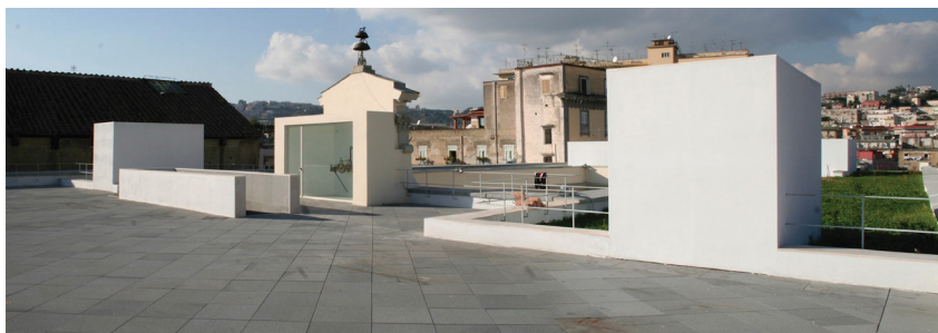
Fig. 4. The building's roof, Palazzo Donnaregina, Naples (Laura De Riso, 2025)
