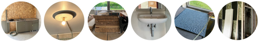
Fig. 8. Reused materials: kitchen, lighting fixtures, Fontex panels, sanitary appliances, carpet tiles, insulation (MAKER architecten)
