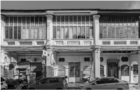
Fig. 2. A row of shophouse in George Town, Penang, with a coffee shop, a residential, and an office on the ground floor (author, 2023)
