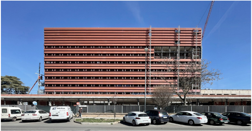
Fig. 1. Ciudad Real, Administrative Headquarters, under construction 2024
