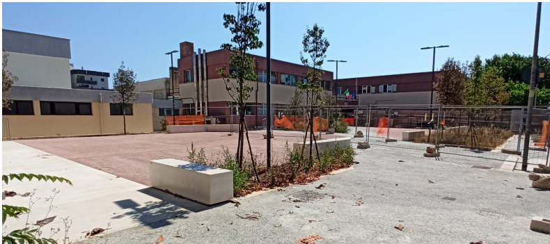
Fig. 4. The square under construction with the school in the background (Mariella Annese, 2025)
